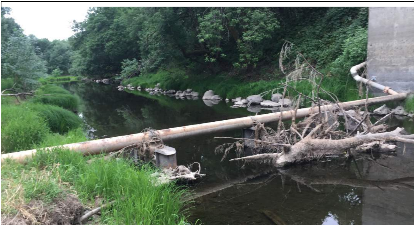
Above: View west of the pump station, suspended pipe, and steel piling to be removed. July 19, 2018.
