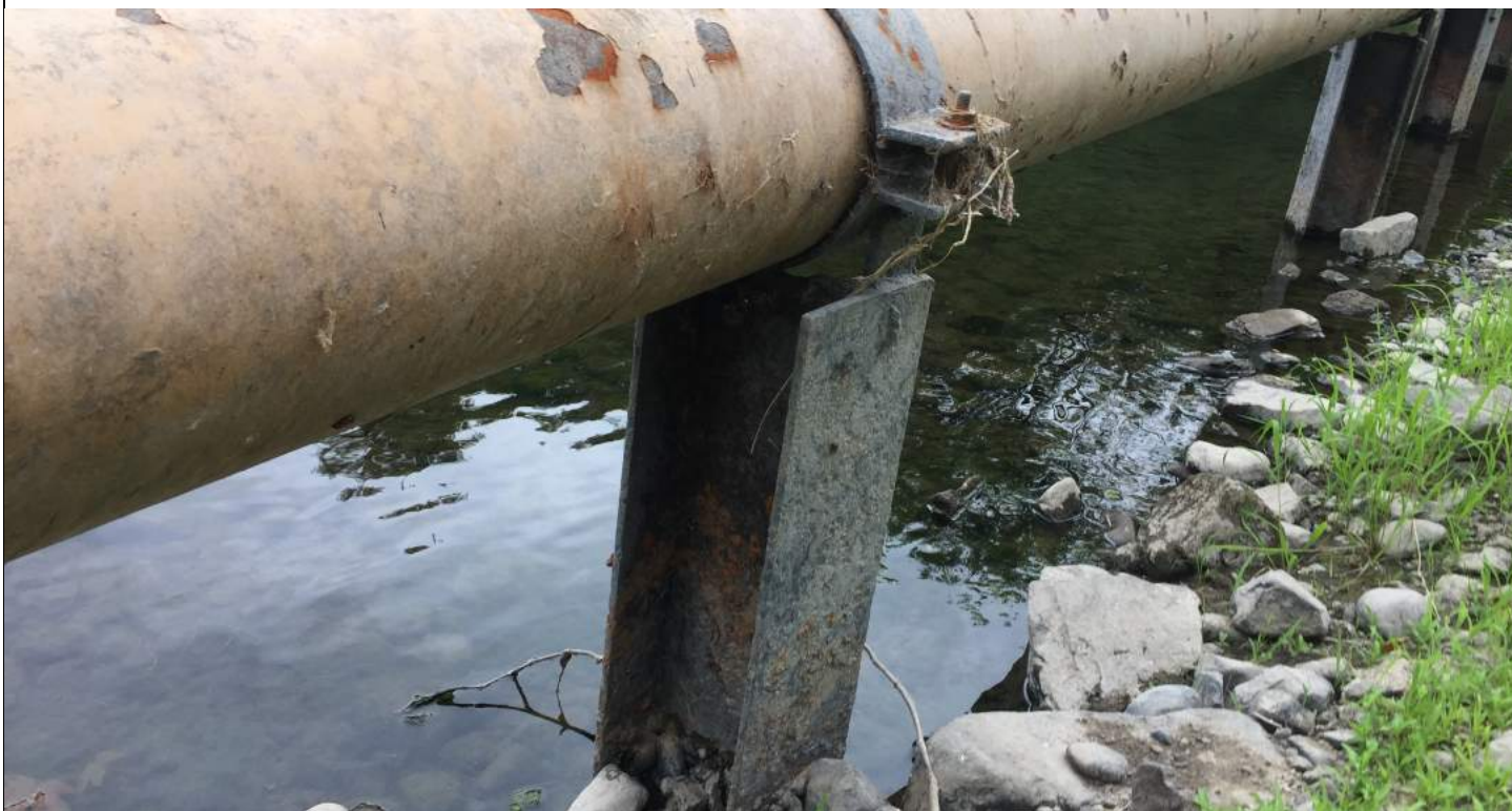
Below: Close up of suspended pipe and steel piling to be removed. July 19, 2018.
