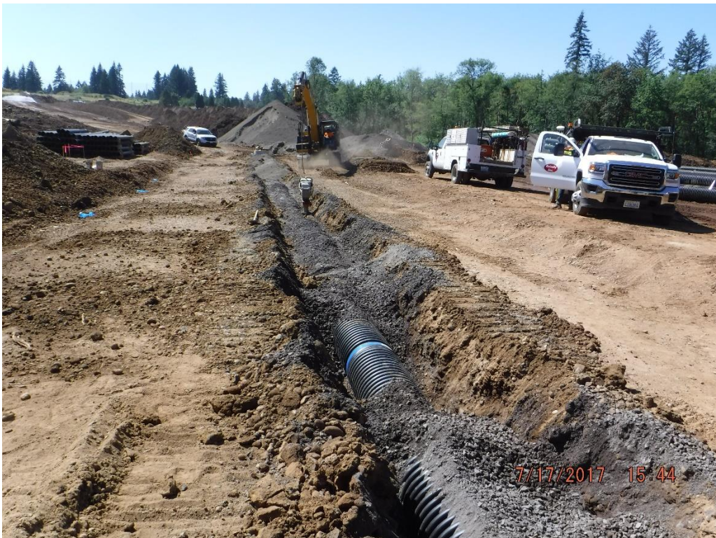
Camas Meadows Drive Storm Main Line Installation by Developer.
