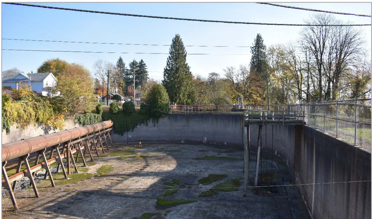
Figure 6. Existing Clarifier Tank
