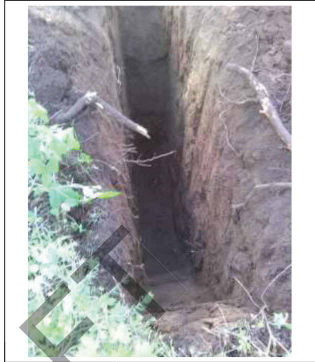
Dry, sandy soils to 16 feet in TP-12
