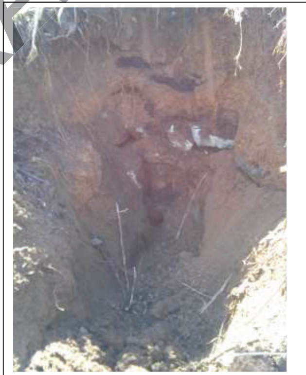
Unconsolidated fill material in TP-8
