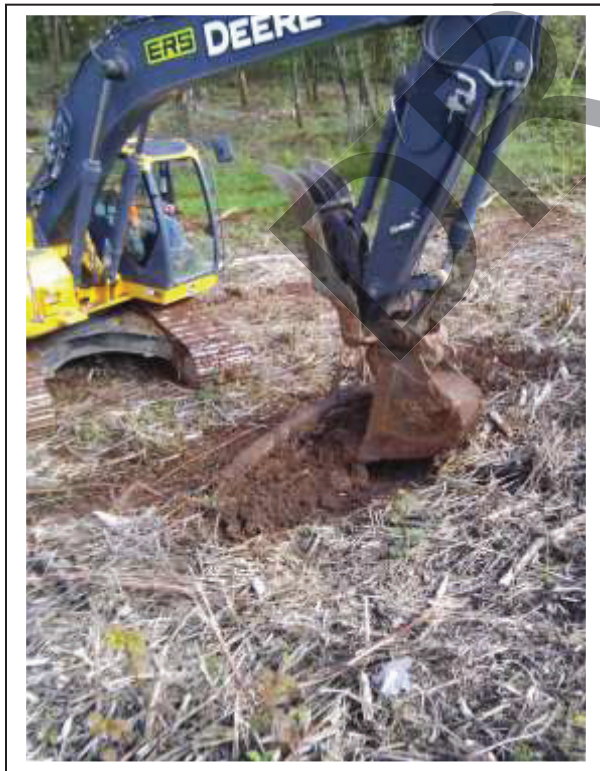
Exploring unconsolidated fill material in TP-8
