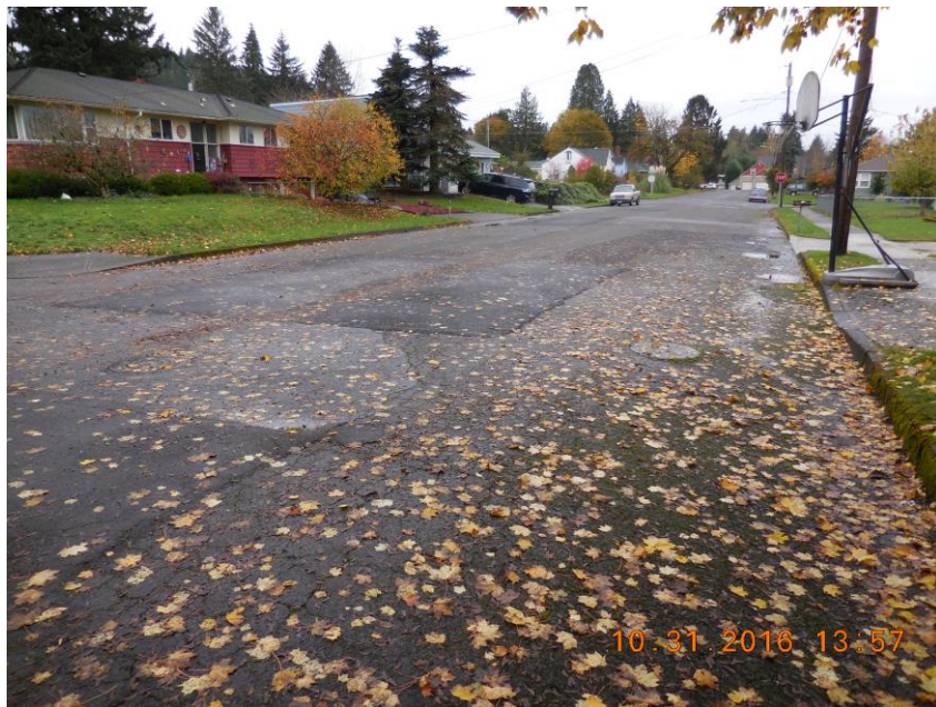
Figure 3 Dallas St. looking North
