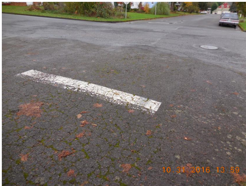
Figure 1 Dallas St. looking North
