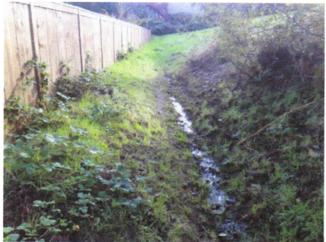
Drainage ditch at eastern edge of site
