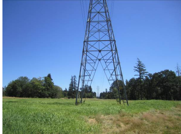
Typical view powerlines (to the south)
