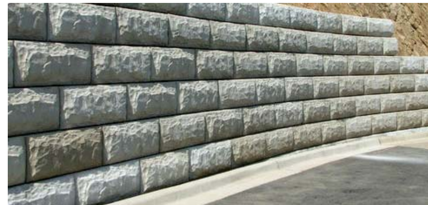
RETAINING WALL BETWEEN UPPER AND LOWER PROPERTIES
